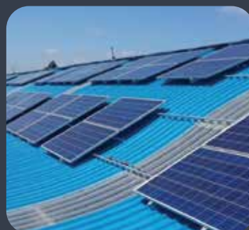
TIN SHED MOUNTING STRUCTURE:
