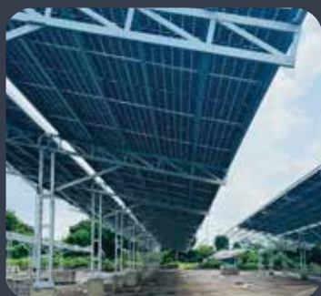
CAR PARKING STRUCTURE
