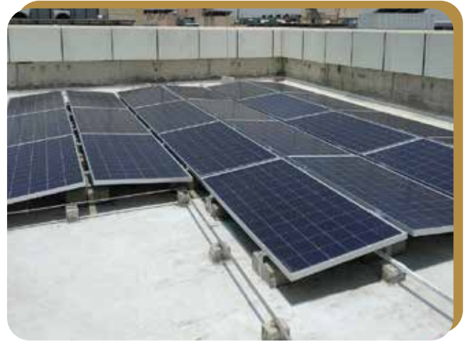
Low Ballast Structure
